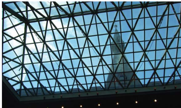
Glass atrium over courtyard.
