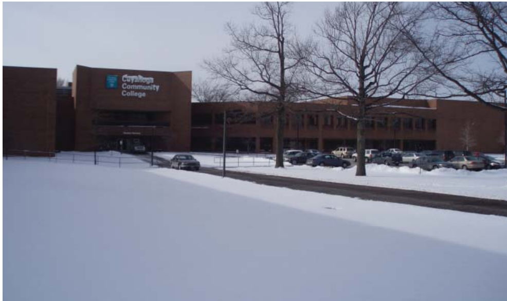
Unique Building Entrances. The distinctive "winged" entries can be reinforced by creating a landscaped courtyard setting at these locations, particularly on the east side facing York Road.
