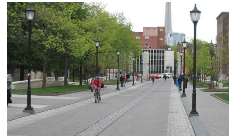
Secondary pedestrian-priority roads should force vehicles to proceed slowly. Distinctive paving indicates pedestrian crossing areas.
