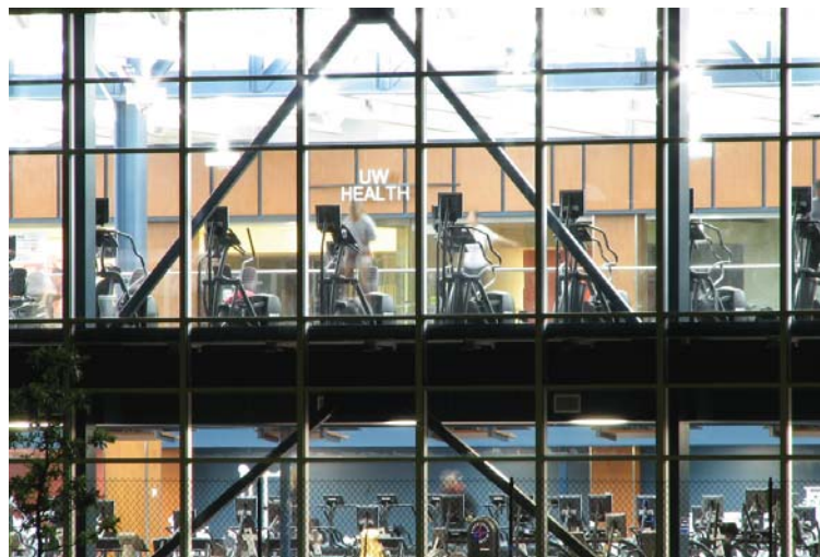
Glass facade brings life to the street from inside fitness areas.
