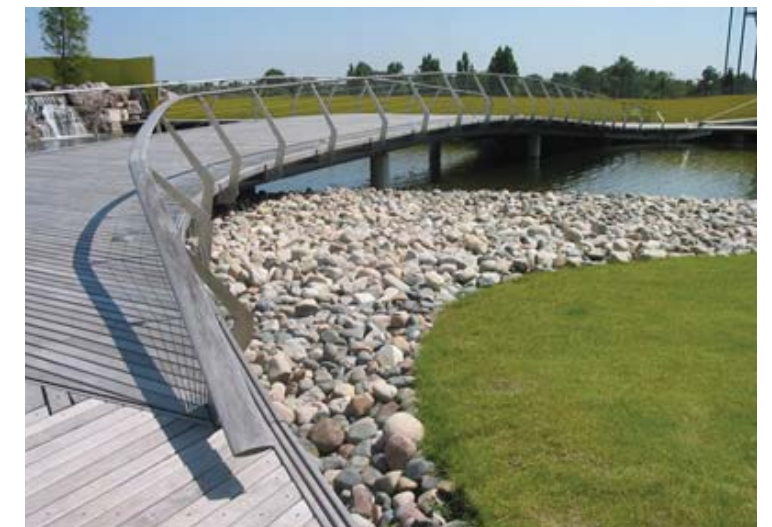
Paths should connect to features that allow users to experience the water, such as modern bridges.
