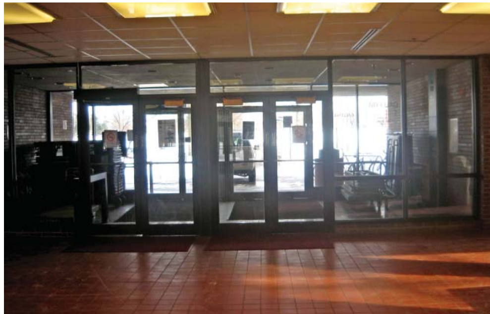
Undistinguished Facility Entrances. The campus lacks a hierarchy of entrances that indicate where important and frequently used places are located.
