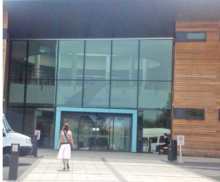
The demolition of EEC creates an opportunity to make a new welcoming entrance to ELA. Extensive use of glazing and decorative paving creates a formal entrance area.
