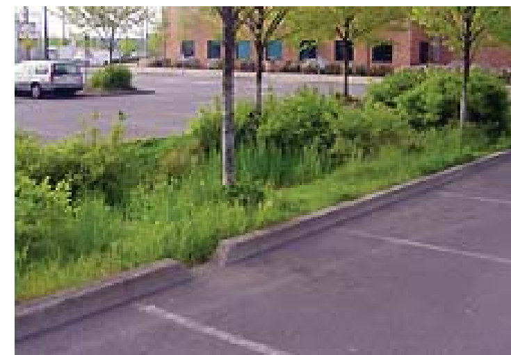
Bioswales filter stormwater runoff from parking areas and allow for local infiltration.
