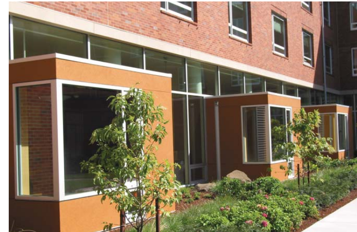
Landscaping along the edge of the new wing can create an attractive pedestrian realm.
